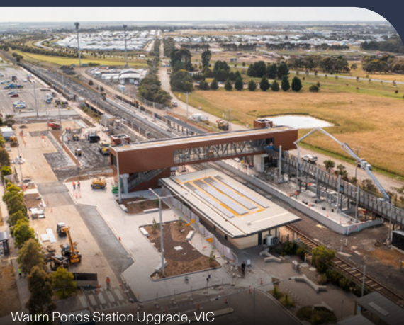
METRONET Yanchep Rail Extension (NEWest Alliance) – Alkimos Station, WA
