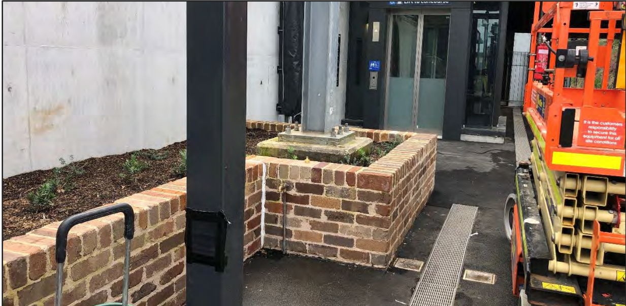
Photo 7. Garden bed located around the north-eastern end of the Platform 1 drainage system. Date: 21 April 2023.
