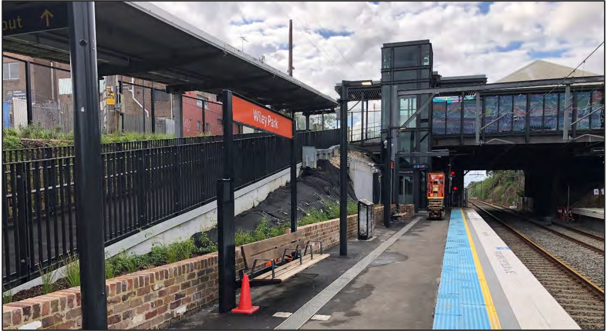
Photo 5. General current condition of Platform 1, Wiley Park Station. Date: 21 April 2023.
