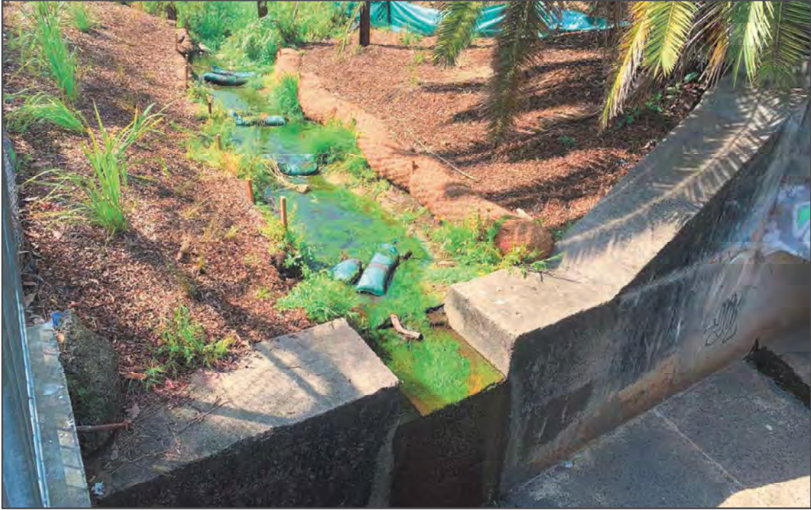
Photograph 3. Condition observed from downstream discharge point WP2-DP1 that was located within the rail corridor and immediately upstream / south from WP2 during the monitoring event. Significant algae growth was observed at this location at the time of monitoring – 15 September 2023.
