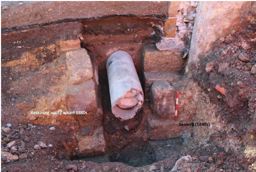
Photo 3 1840s seawall and 1880s retaining wall uncovered at Balmain East, 2016
