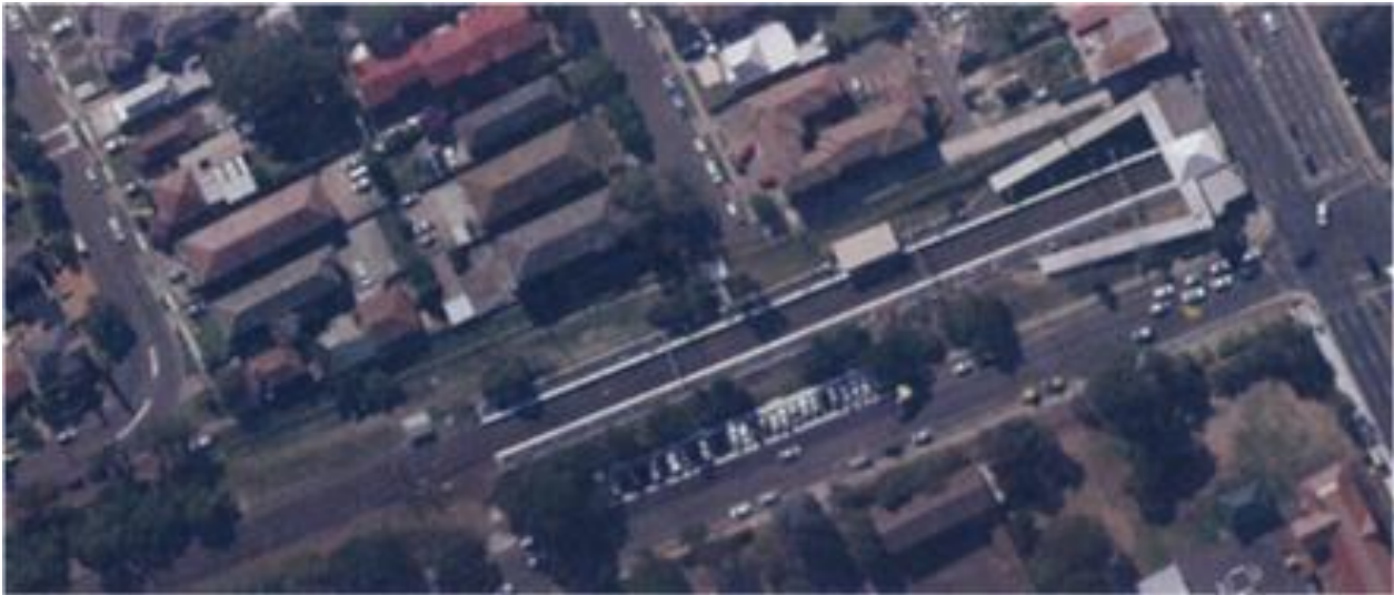
Figure 6 6.1.2.3 Wiley Park Station
