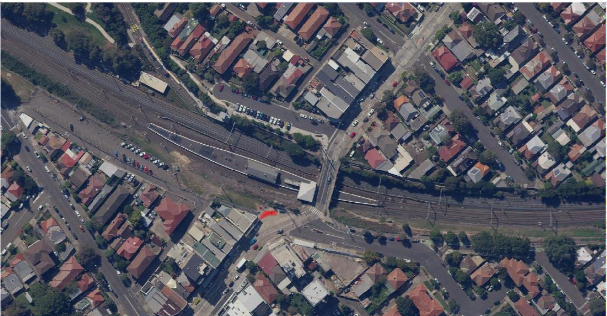
Figure 12 Dulwich Hill Station- Wardell Road, car park space (1 No), No interference to bus stop
